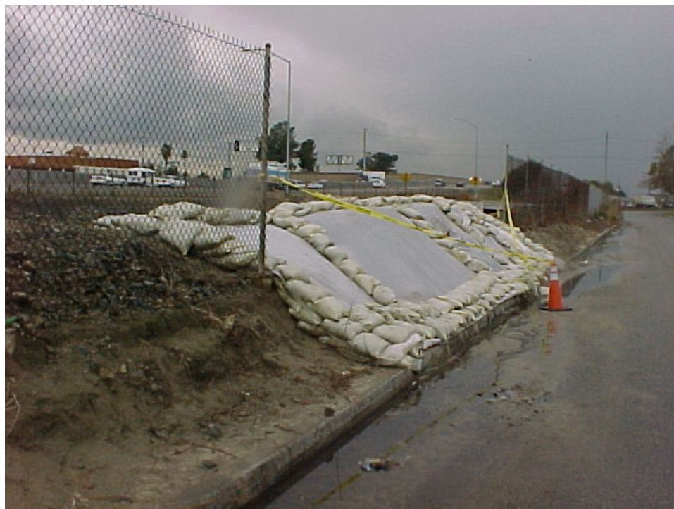
B01 U/S 91 freeway at Burton way (side view)
