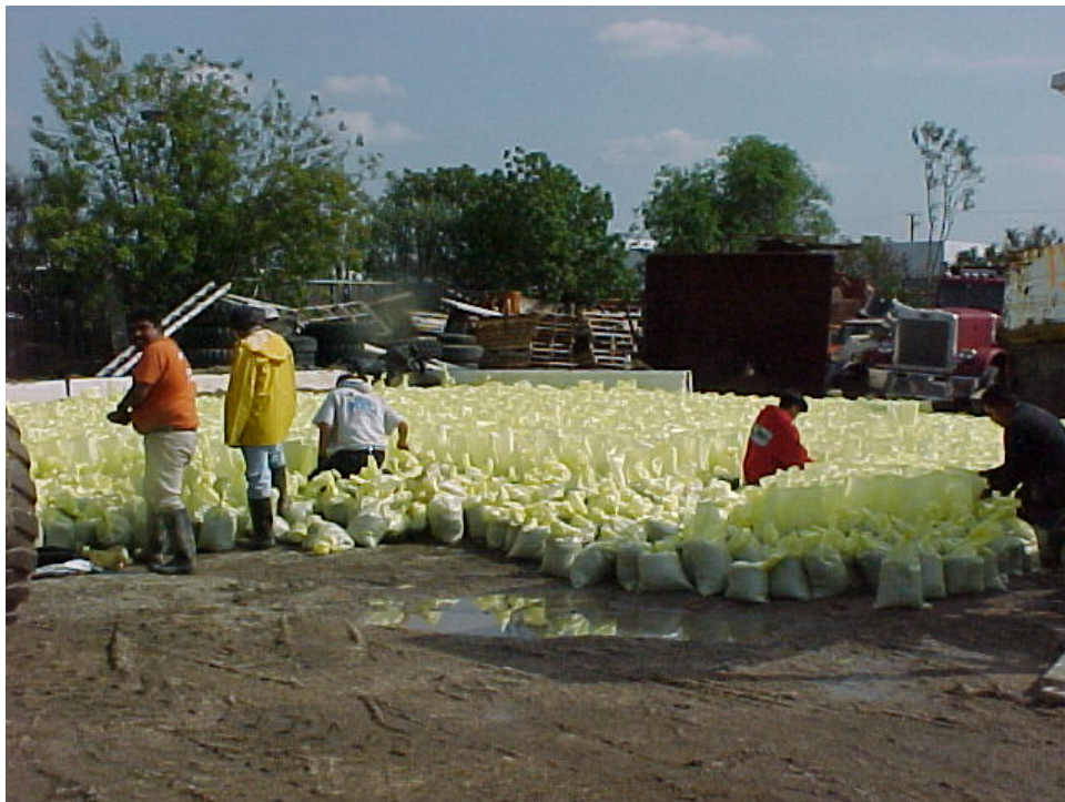
Bags are filled then loaded onto trucks and transported to job sites
