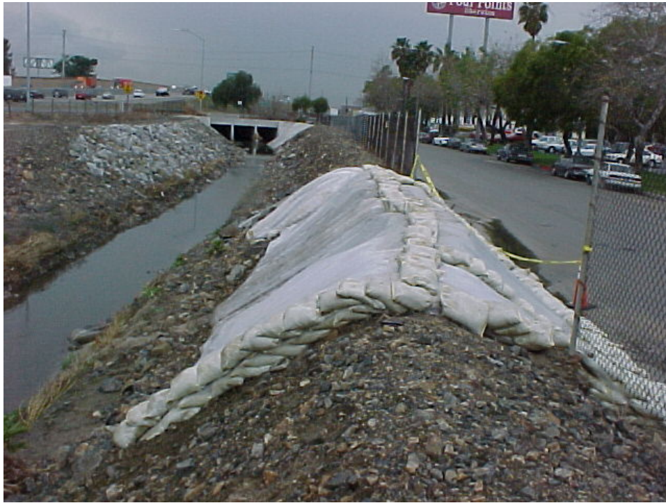
B01 U/S 91 freeway at Burton way (top view)
