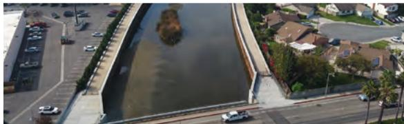
East Garden Grove-Wintersburg Channel and Ocean View Channel system is one of the underlying channel systems that does not currently have the capacity to contain the 100-year flood as the channel banks and levees have over-topped at several locations.
