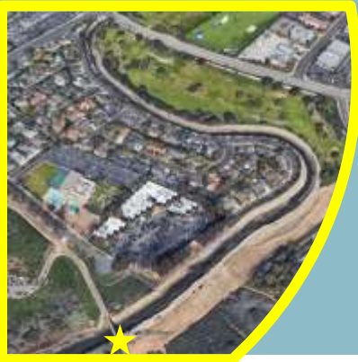
SANTA ANA-DELHI CHANNEL IMPROVEMENTS
