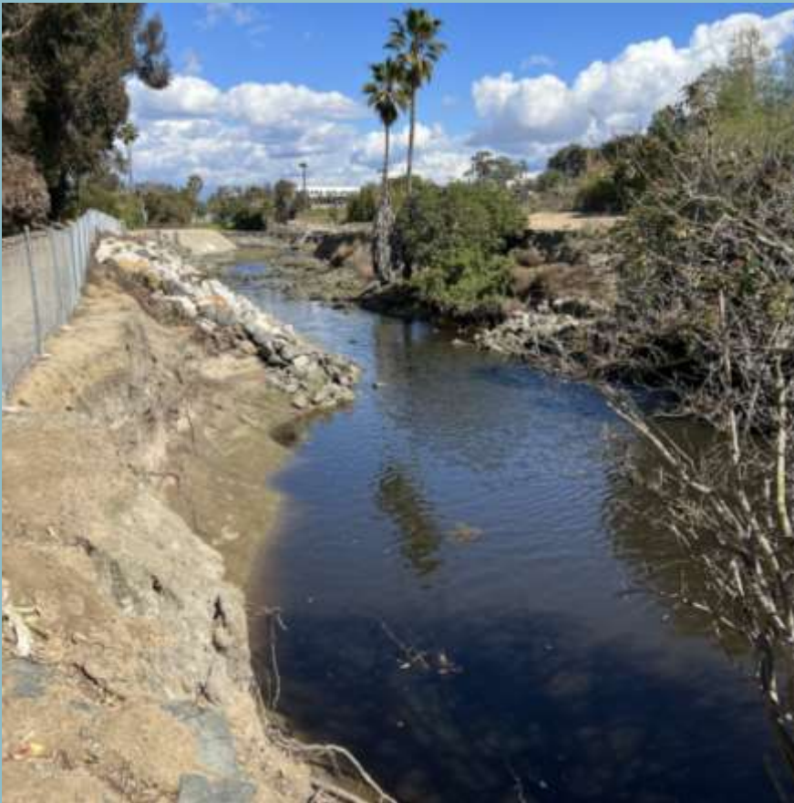
Lower Reach (West Side)
