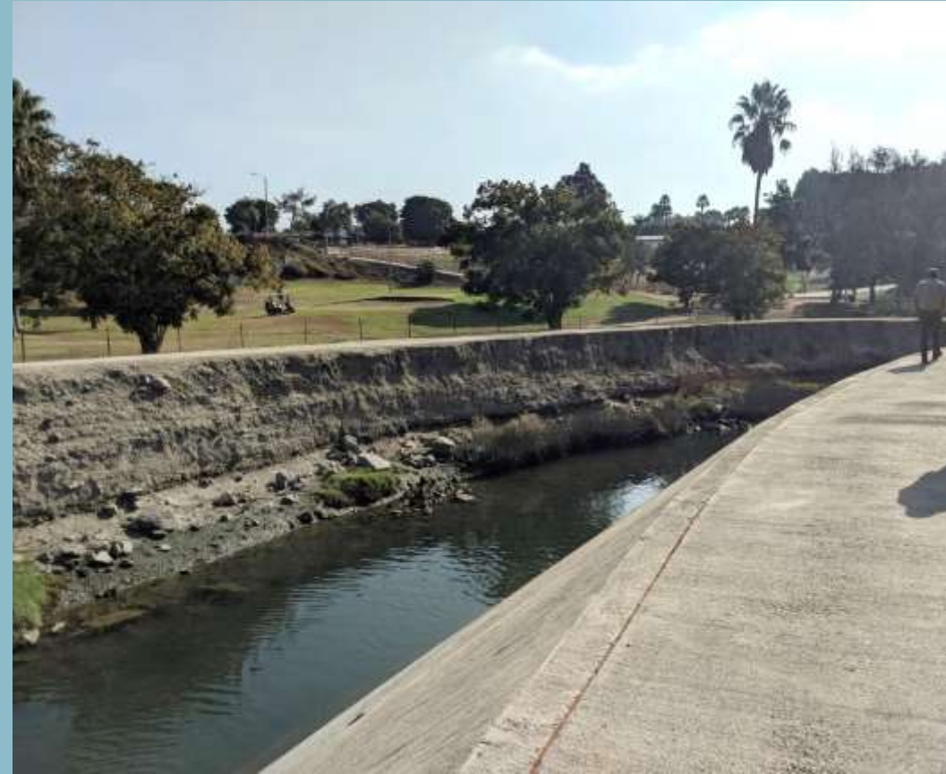
Upper Reach (East Side)
