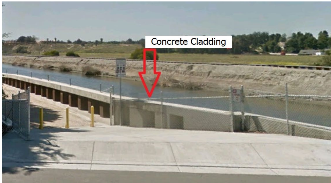
Figure 12-2: Concrete Cladding on Sheet Piles
