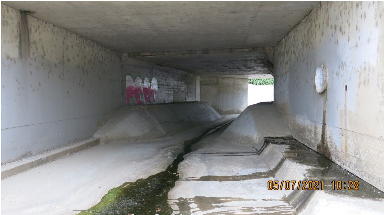
Figure 6-1: Abrupt Curve Re-alignment with a Constriction (Brea Creek Channel (A02) at Beach Blvd)
