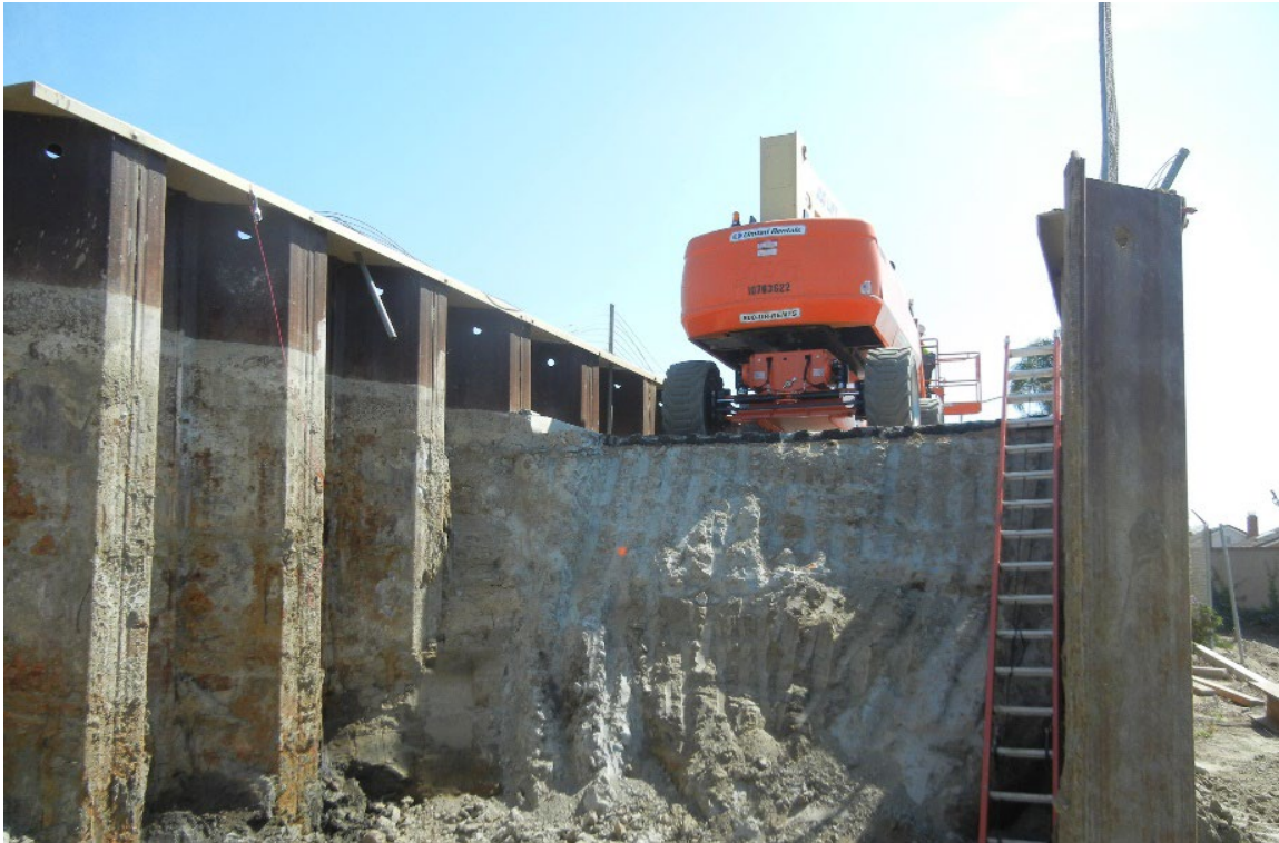
Figure 11-5: Construction Equipment atop DSCM
