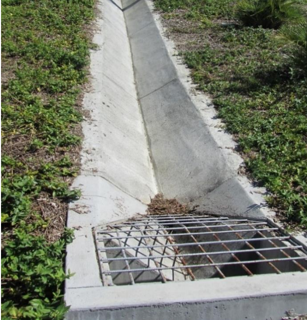
Figure 6-3: Down Drain Example
