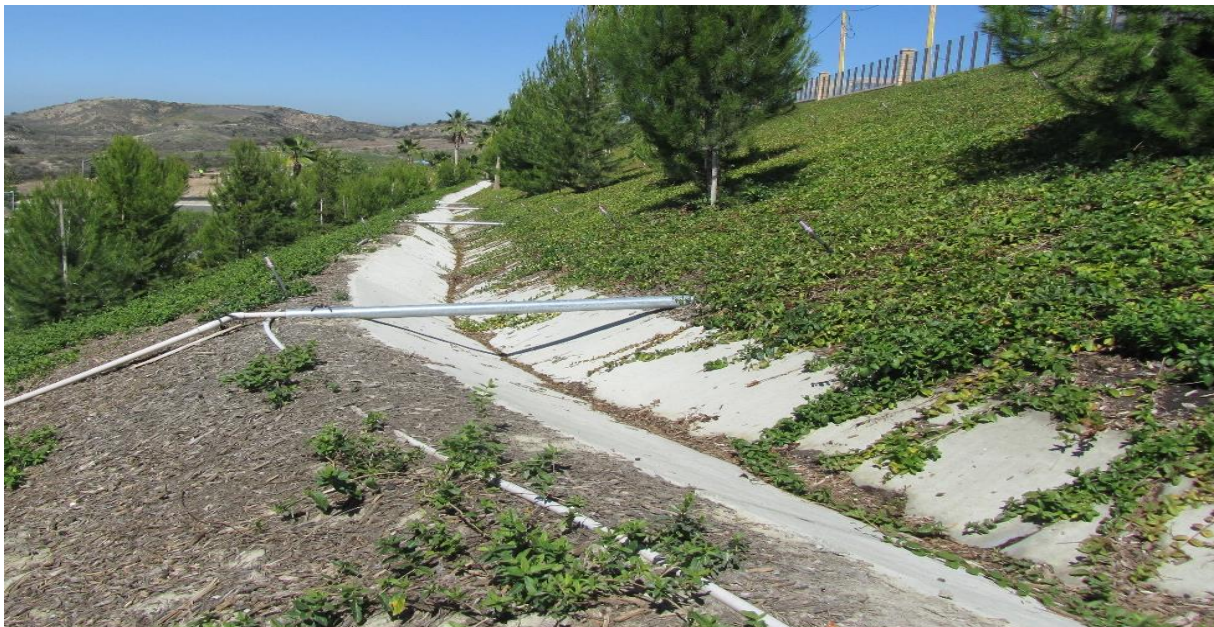
Figure 6-2: Terrace Drain Example
