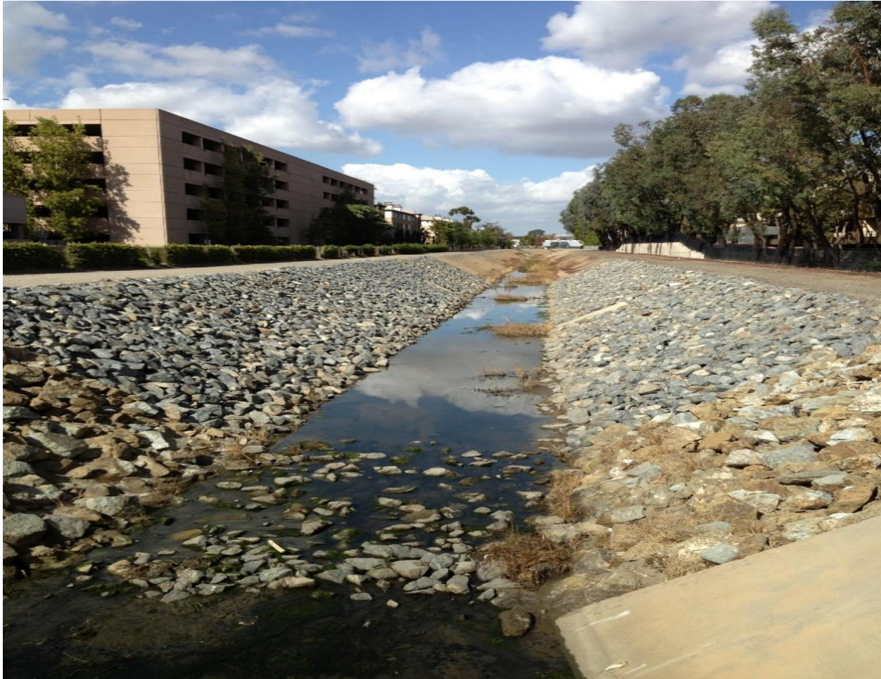
Figure 6-5: Rock Riprap Channel Example
