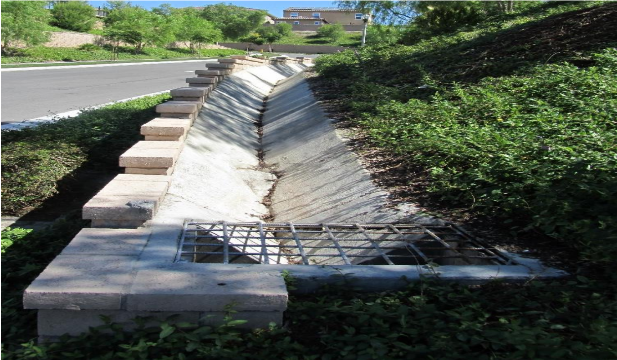
Figure 6-4: V-ditch Example
