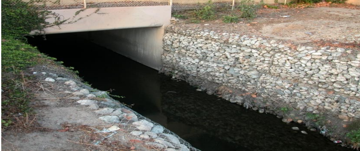
Figure 6-6: Gabion Channel Lining Example
