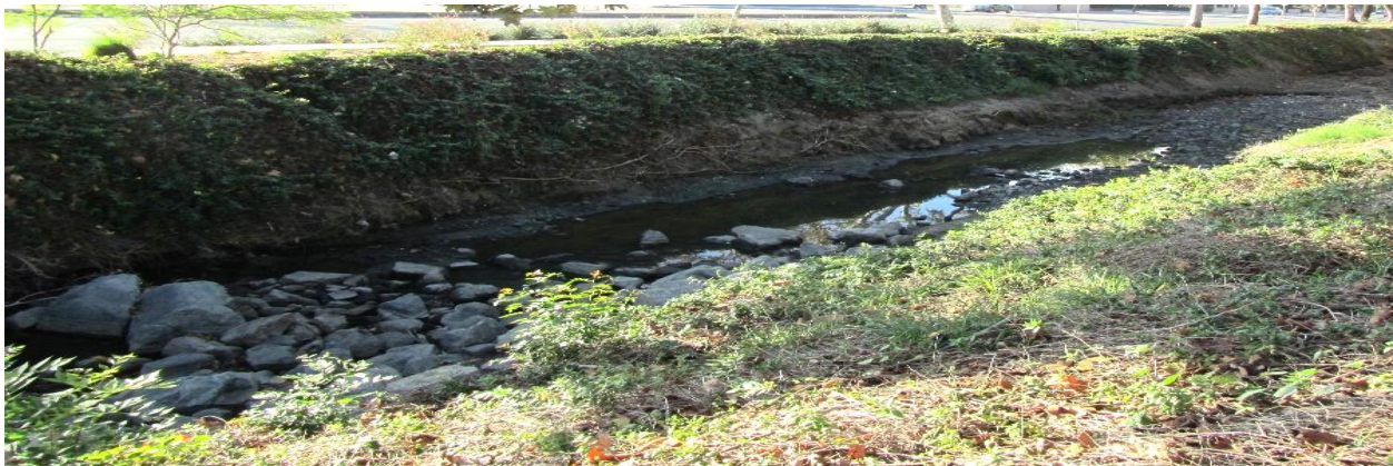
Figure 6-7: Vegetated Channel Example
