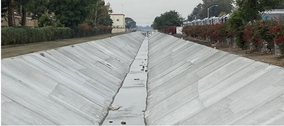
Figure 6-1: Concrete Lined Channel Example
