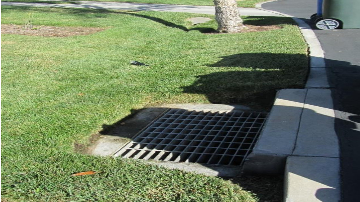
Figure 6-9: Water Quality Vegetated Swale Example
